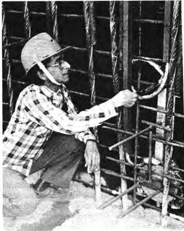
Fig. 3.29.1. Pressure Cell Assembly in Position before Concreting<sup>169</sup>
